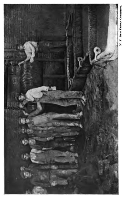
Unguarded Vata in Wire Factory. The Vata, almost Level with the Floor, Contain Sulphuric Acid and Scalding Hot Water.
